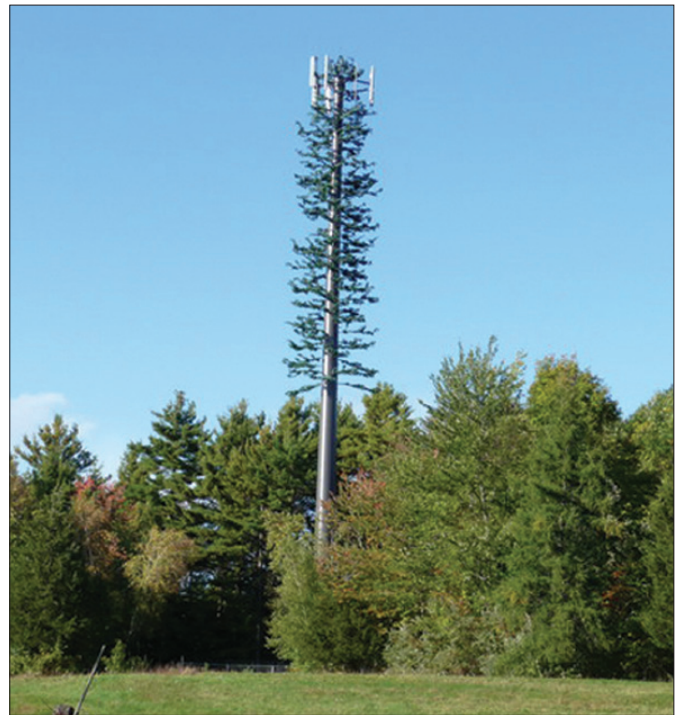
Towers come in a variety of shapes and sizes, including steel lattice towers, guyed wire towers, tubular poles and stealth structures such as fake trees and flagpoles.
