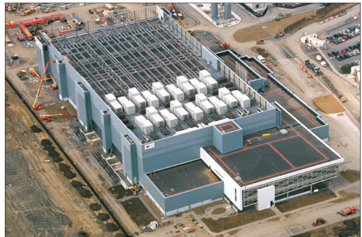
AN AERIAL view of Microsoft’s data center in Dublin, Ireland
